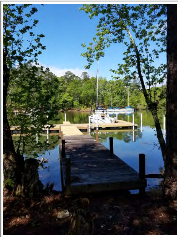
Dock A view
